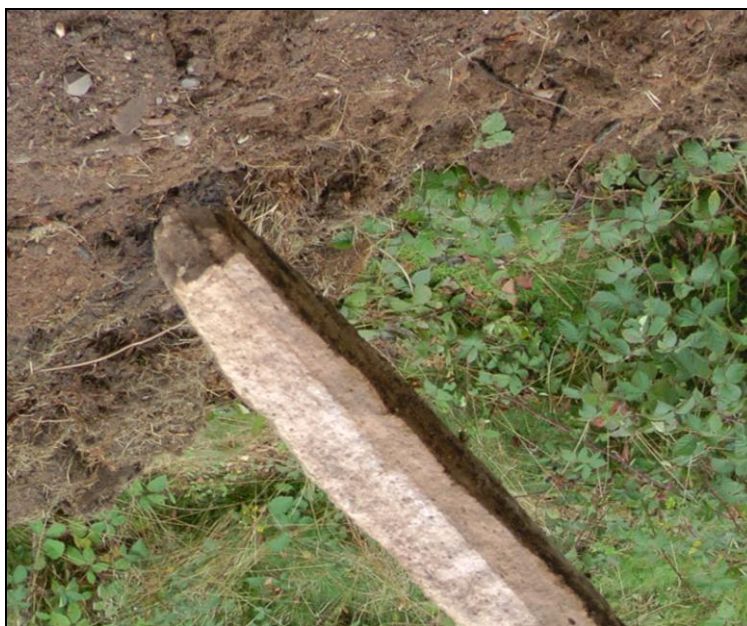
Plate 6 Section of concrete super structure showing both layers
